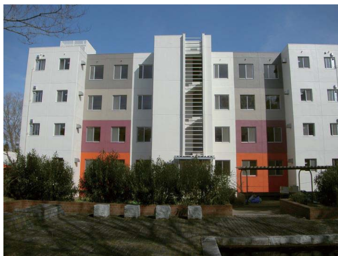
Hirasuna Student Residence Hall
