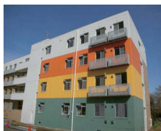
Renovated Building (Hirasuna#1)
