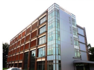
Building of Innovation Medical Research Institute
