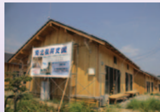
Temporary compound designed by our teacher (Iwaki City)
